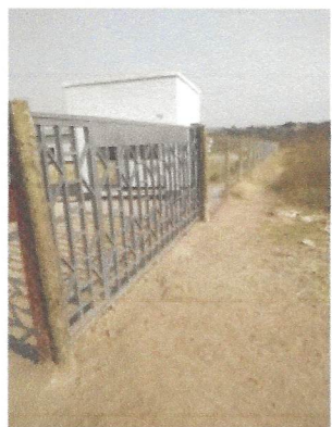
Gate House & Access Gates to The Mulyata site
