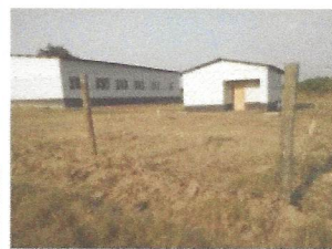
Fenced feeding station & toilet block (previously funded by Radio Cracker)
