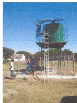
Secured Borehole site
