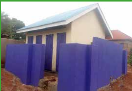
New Latrine Block
