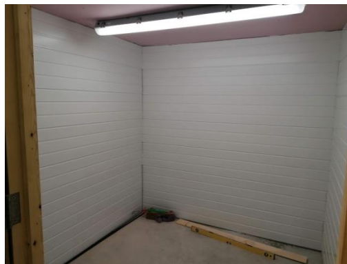
The new disabled toilet facilities – work still in progress
