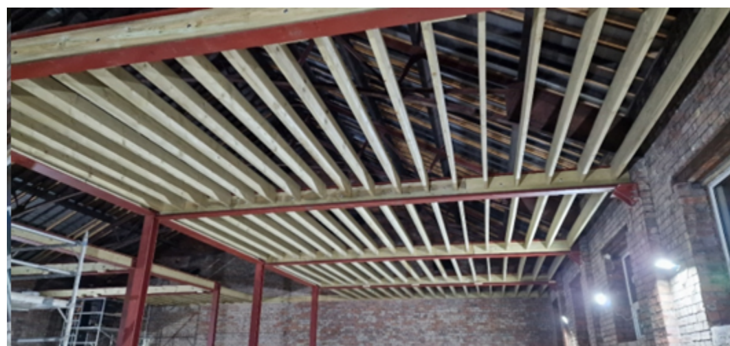
Steels installed and floor construction started.
