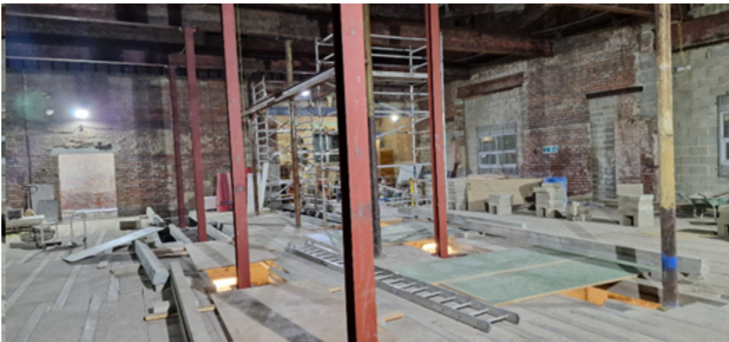
Basement footings dug out and steels installed.
