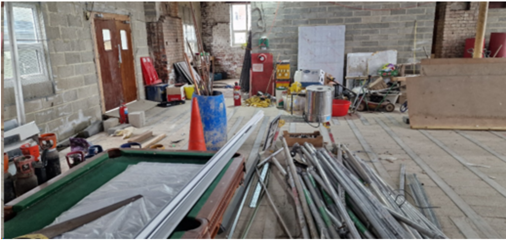
Clean-up operation at 92 Lady Pit Lane (Flats Project)
