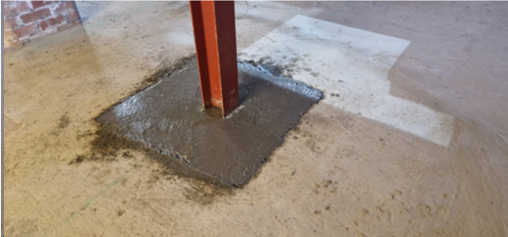
Basement footings dug out and steels installed.
