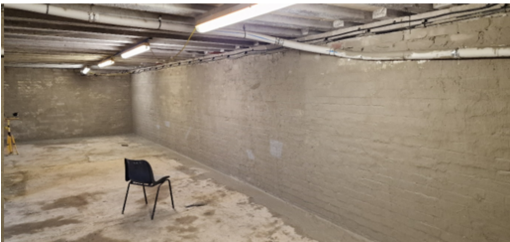
Basement waterproof tanking complete
