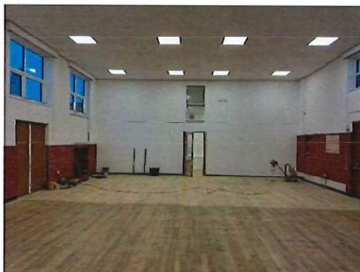
Floor being sanded, sealed, and varnished.
