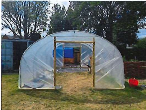
Second polytunnel – finish and fit out underway!
