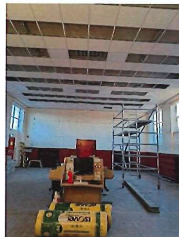
New ceiling and LED lights going in, raised corner removed
