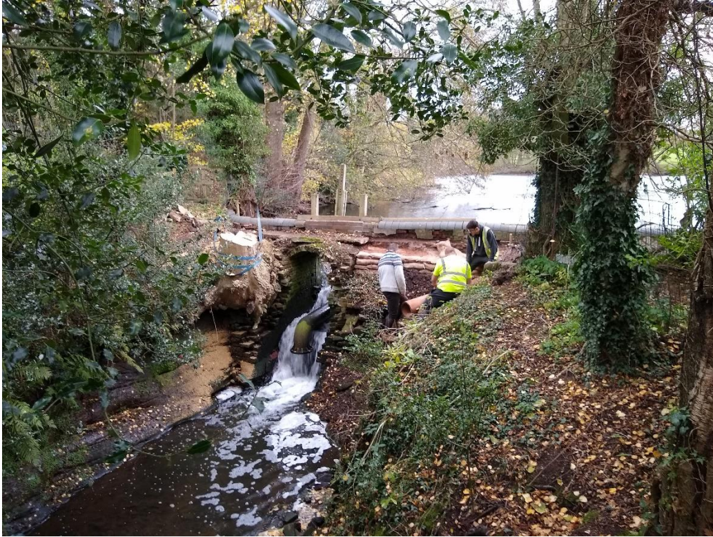
Pool spillway at start of repair work
