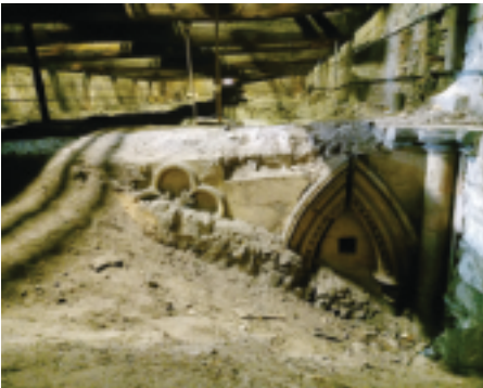
East tower base north side
