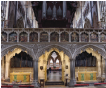
Exeter cathedral pulpitum showing the four Purbeck marble piers supplied by William Canon of Corfe in 1319
