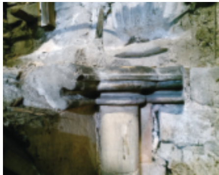
Purbeck marble moulding on ruined west side of eastern crossing north side
