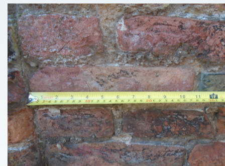
Fig 8 'Long' brick. Reused example from rebuilt wall in Friars Lane
