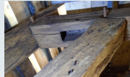
Fig 7 Carpenter's mark and reused timber
