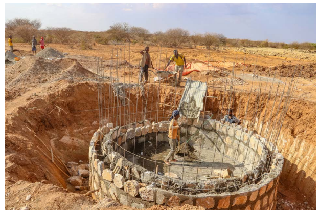
The building of a dam in Hargalle, Ethiopia as part of a project to support 3,000 farming families affected by drought
