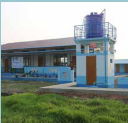
A school in Kan Chaung village, Myanmar, renovated by Islamic Relief this year. We added three classrooms, toilets and new school furniture. Safe drinking water and a new entrance road were also provided, supporting children to continue their learning in a safe and suitable setting.
