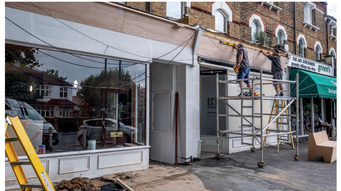
Renovation of Redemption Roasters
