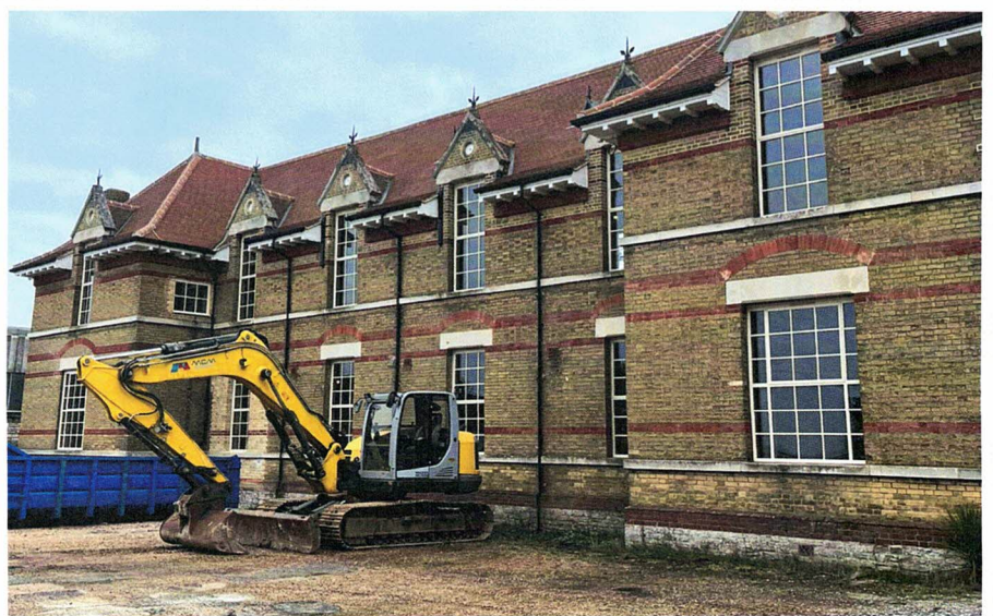
Building works at Victoria Barracks
