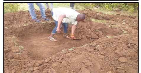
Digging shallow tanks
