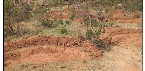
Shaping earth bunds
