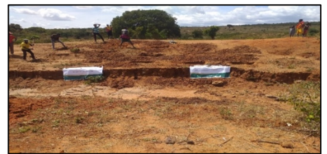
Constructing staggered trenches
