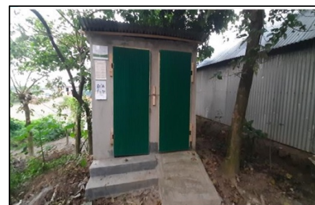
A toilet facility in Narayanganj
