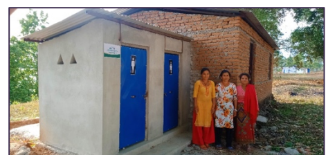
Community toilet blocks
