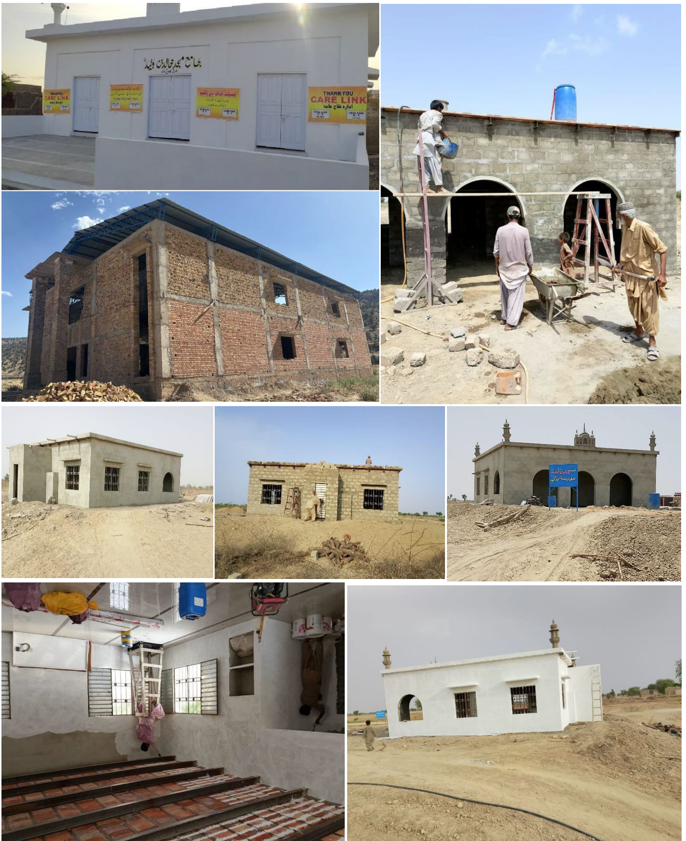
Figure 10: Community Centre Construction
