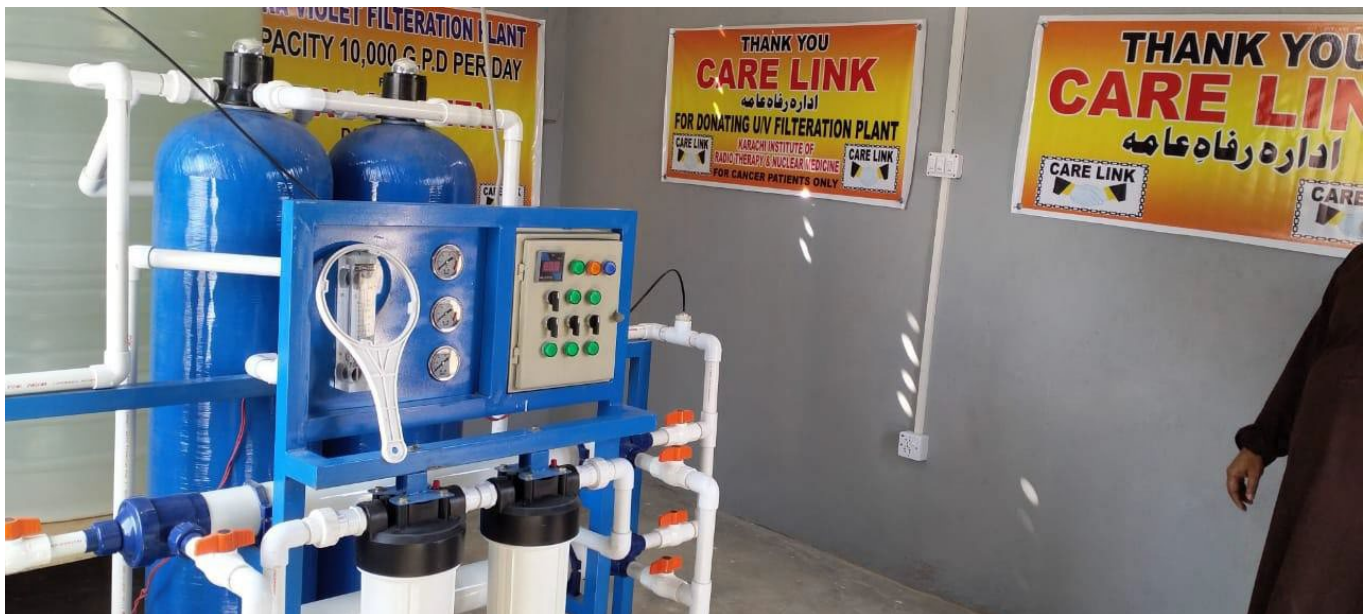
Figure 2: Water Filtration Plant Vinder, Baluchistan.
