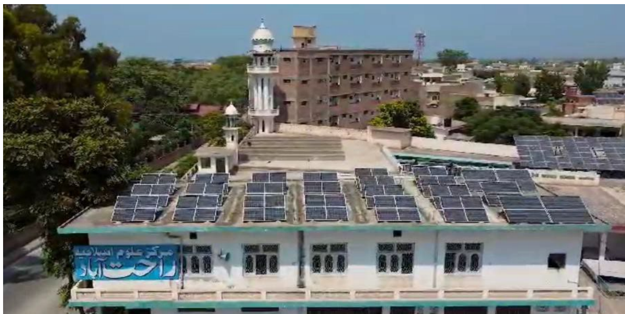
Figure 13: CLT Solar Project
