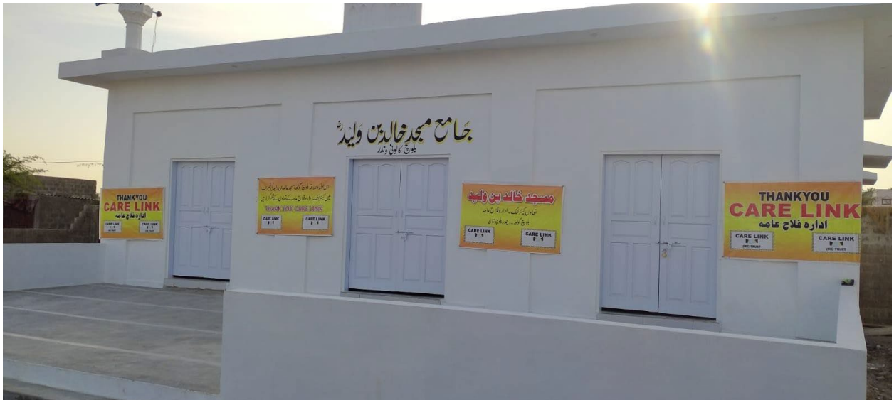
Figure 23:Community welfare Centers for poor communities
