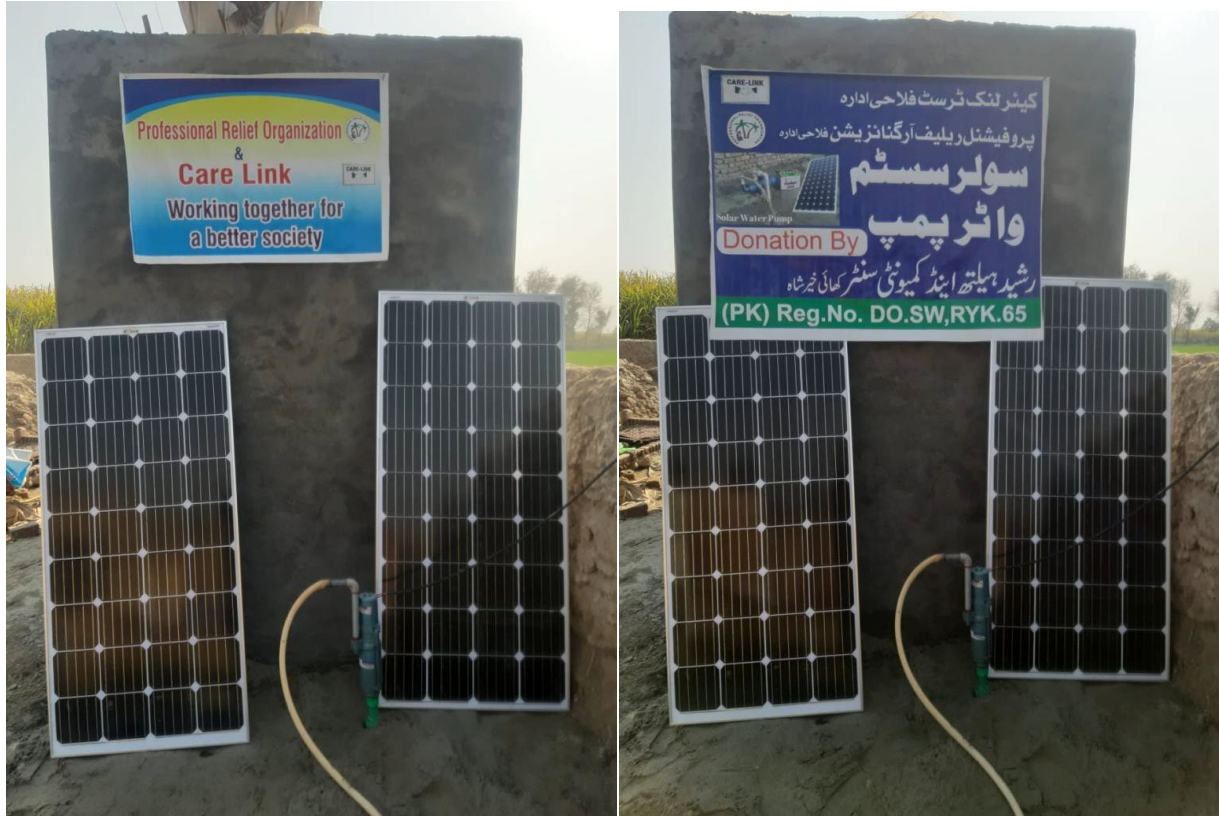
Solar System to support the Provision of drinking water.
