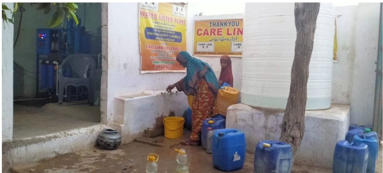
Figure 15: Water Filtration Plant in Balochistan, Pakistan
