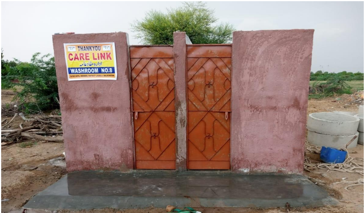
12 Washrooms and toilets built for poor communities.
