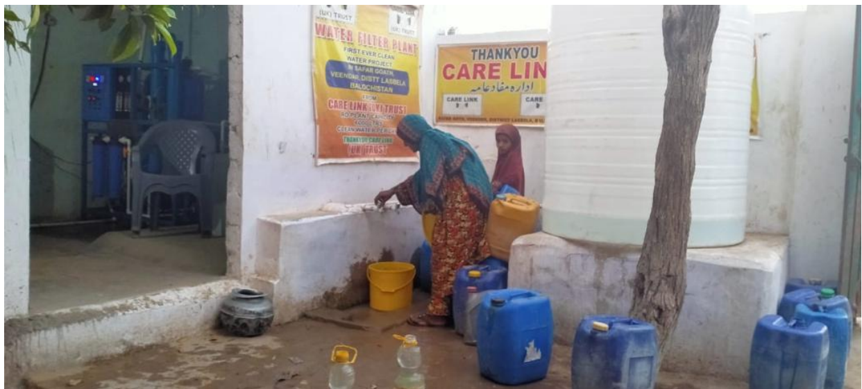
Figure 3: Water Filtration Plant in Balochistan, Pakistan
