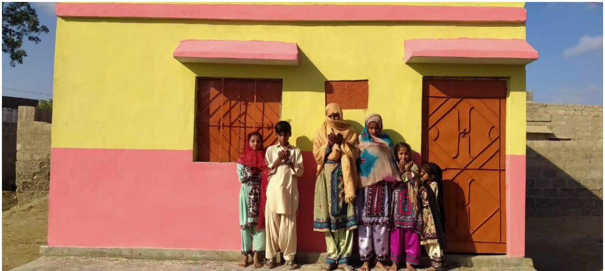
House build for poor family in Balochistan
