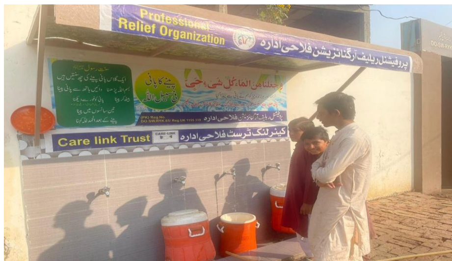
Water Filtration Plant in Khai Khair Shah Village Rahimyar Khan, Pakistan
