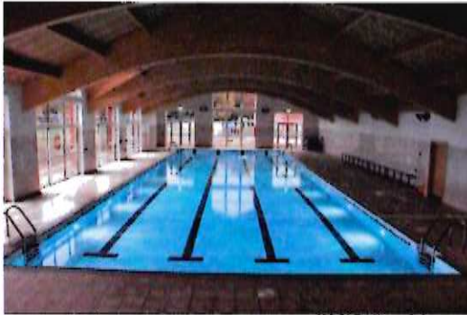
Four Lane Swimming Pool
