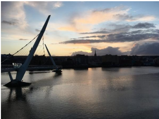
The Peace Bridge – Derry/Londonderry
