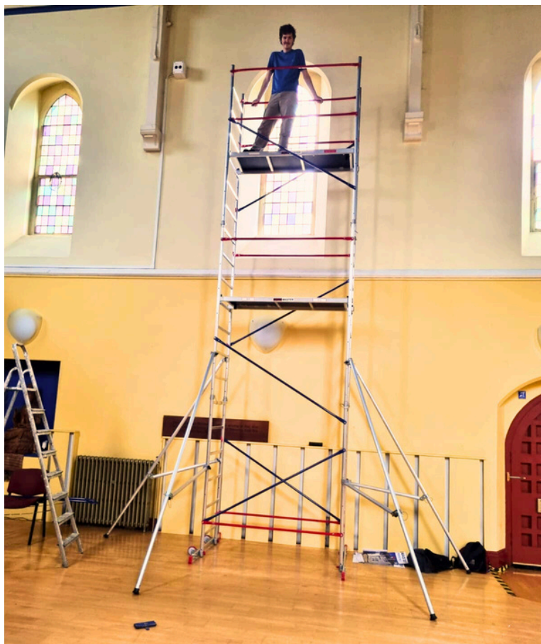
Volunteers prepare for the installation of secondary glazing.
