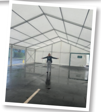
The marquee under construction
