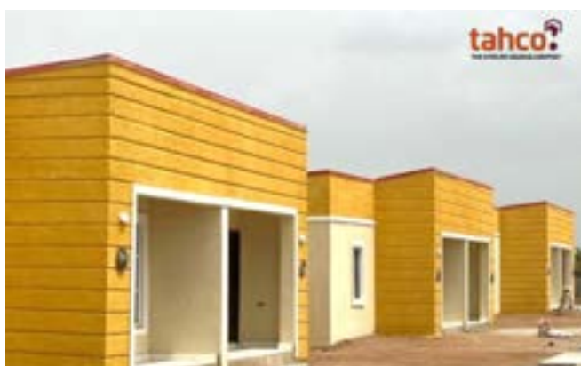
FIGURE 9: THE AFFORDABLE HOUSING COMPANY (TAHC), KUJE
