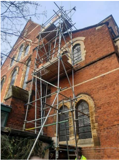
Scaffolds to Chapel South aisle south wall.
