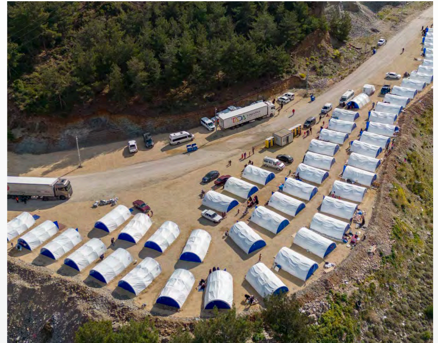
SAMARITAN'S PURSE SHELTER VILLAGE PROVIDED FOR THOSE WHO LOST THEIR HOMES FROM THE EARTHQUAKE
