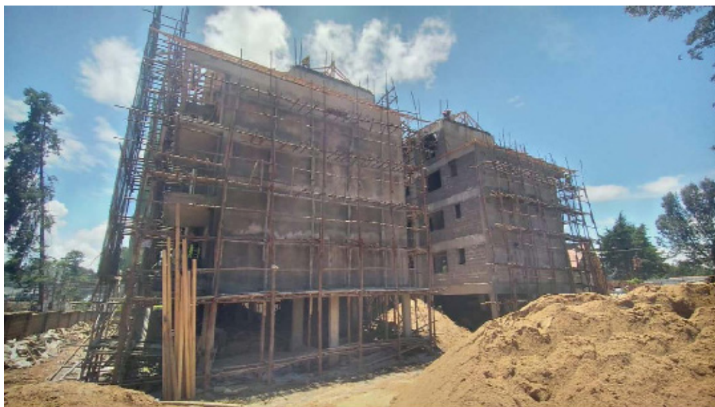
Under construction: new residential units in Nairobi, Kenya
