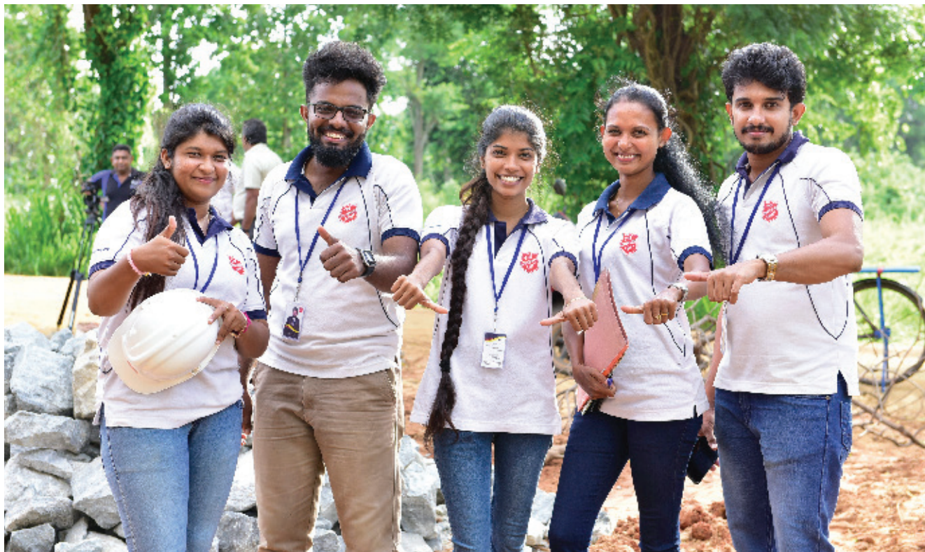
Members of The Salvation Army Safe Water team celebrate the completion of the construction of a well in Anuradhapura, Sri Lanka
