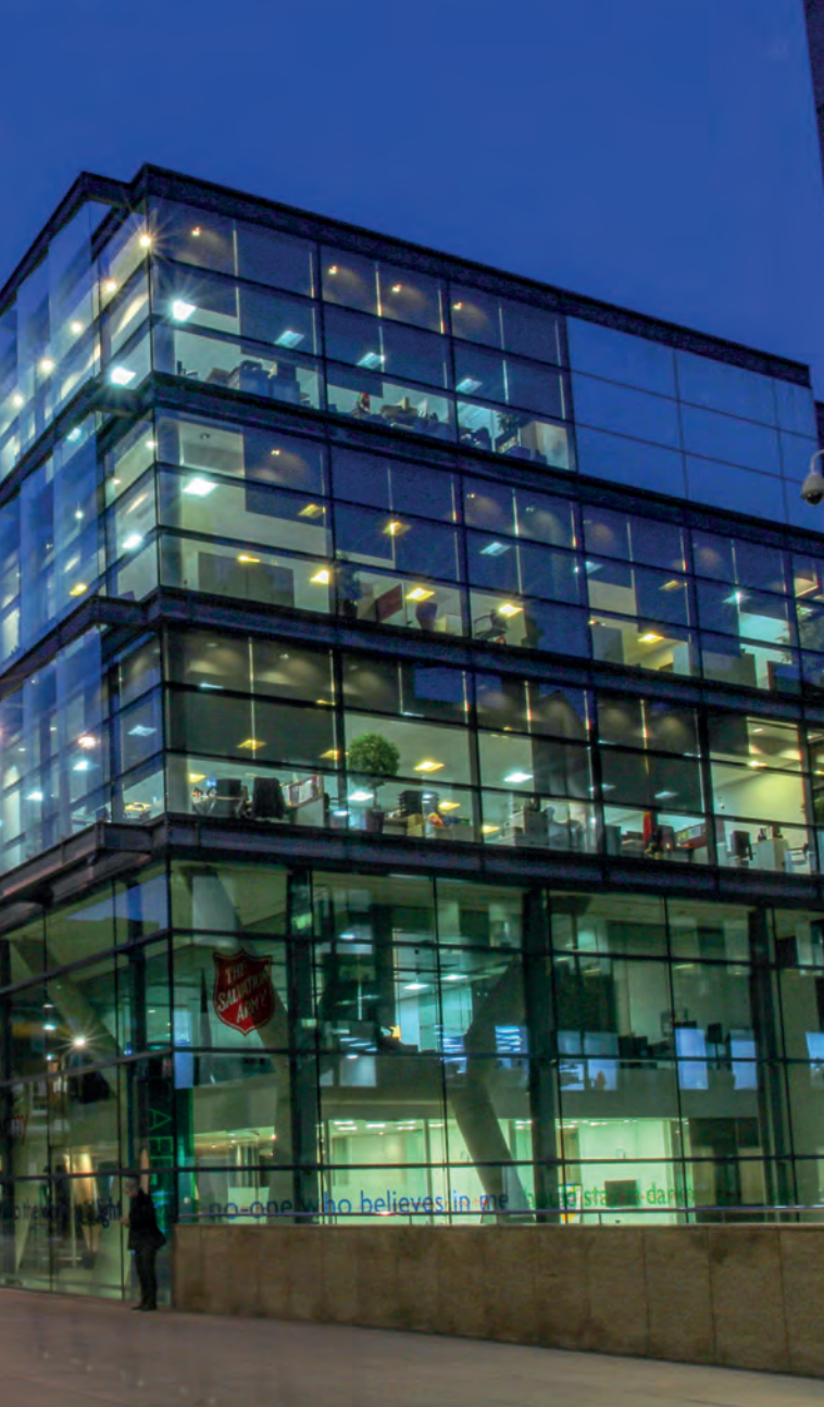
National Headquarters, London, UK with St Paul's Cathedral in the background
