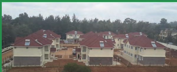
New officer accommodation units in Nairobi, Kenya
